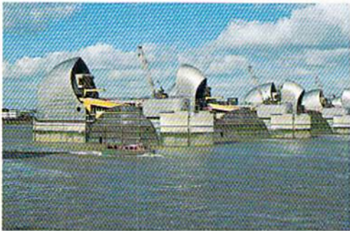
In Tokyo, firemen drill at a specially built apartment complex that serves as both housing and a firewall (top). To protect central London, which is slowly sinking, moveable gates that lie on the bottom of the Thames can be pulled to a vertical position during flooding (bottom). Mitchell studies how communities like these prepare for potential disasters.
